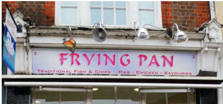
Figure 40 – Unnecessarily extensive lighting.
